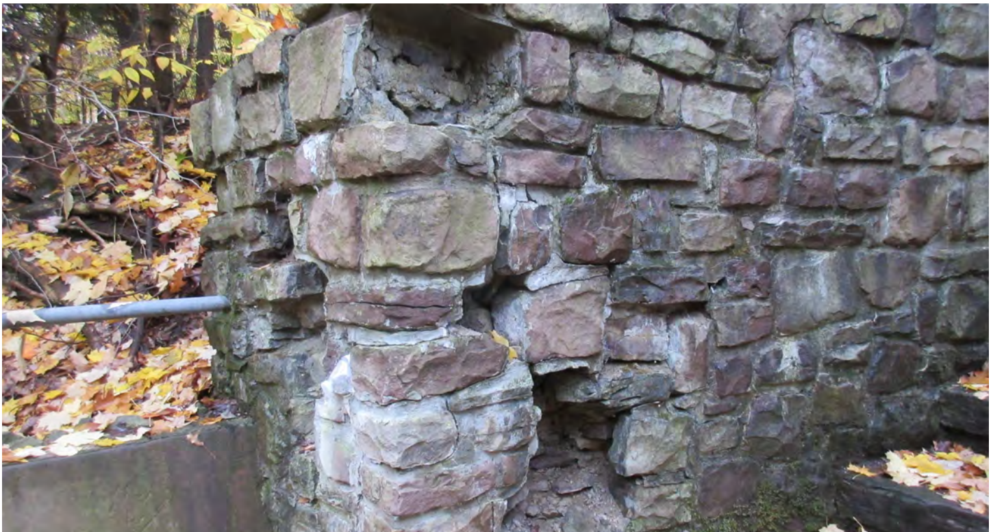
Missing stones and damage observed at the ‘100 steps’
