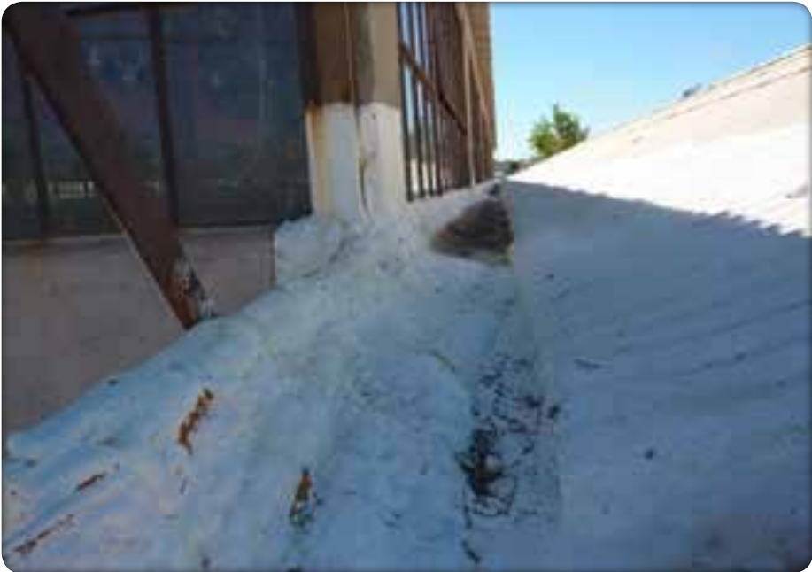
Photo right: View looking south at the gutter between the two sections of the Storehouse. Originally formed from heavy sheet metal, after the gutter developed leaks it was nearly filled with a spray-on foam to seal the leaks.
