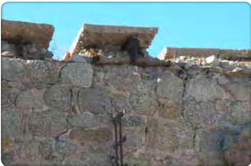
Photo above: In several places the hospital floor slab projects up to, or over, the face of the cell block walls. Diagram Right: Cross section (in black) of the hospital floor slab from the 1994 DWL report. The red rectangle illustrates how a low retaining structure could be added around the perimeter of the slab to keep the aggregate from eroding out from underneath.
