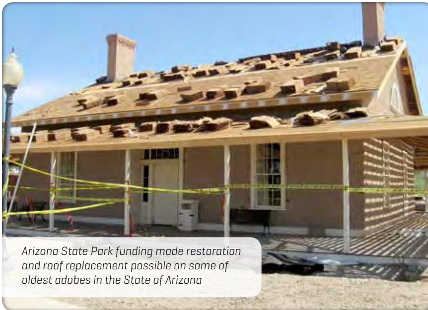
Undergoing a full adobe restoration
